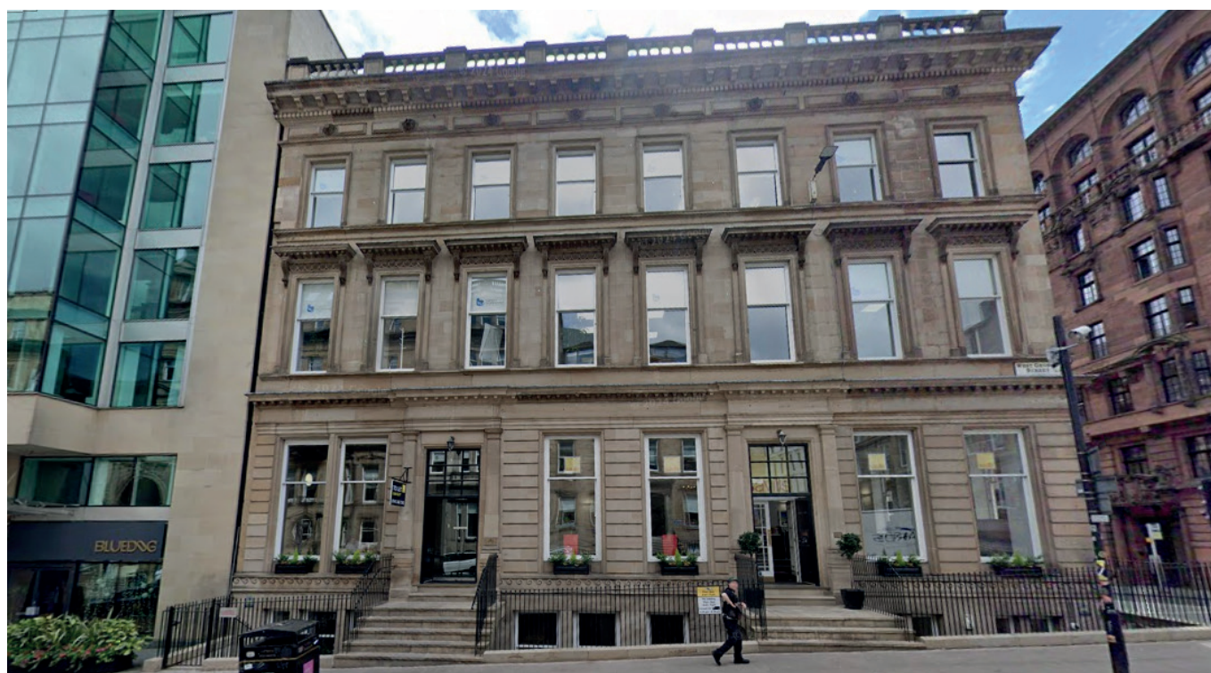
Figure 13: 163 West George Street, Glasgow
